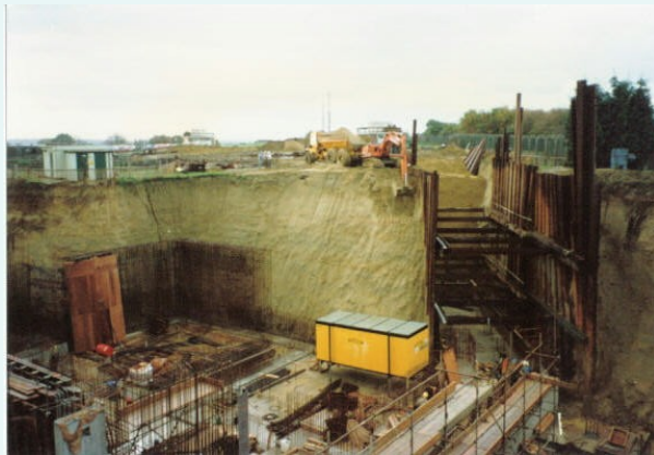
WORKS BEING CARRIED OUT
