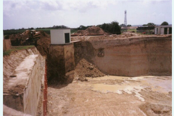
WORKS BEING CARRIED OUT
